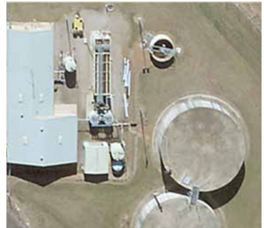
Goomeri Water Treatment Plant
